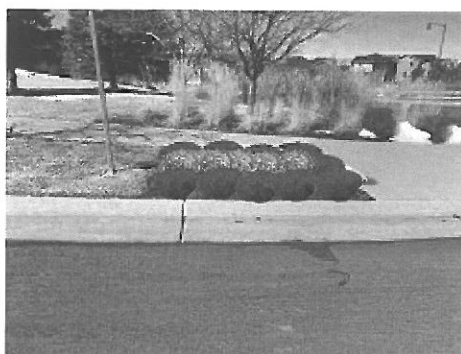
W Side Coolidge ct and Arapahoe
